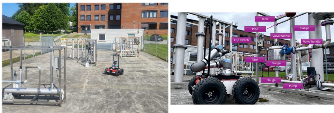
Figure 13. Current status of EQUINOR testbed.
